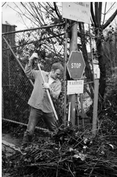
A NOAA crew member helping the neighborhood build a shoreline pathway on Fairview Avenue East
